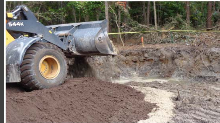
PBA TCRA – Northern portion of excavation during backfilling (8-20-14). Note minimal amount of groundwater in excavation.
