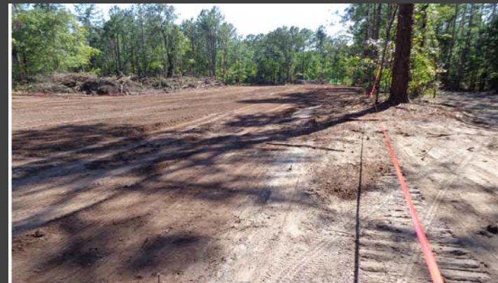
PBA TCRA – Completed backfilled and graded excavation area (8-28-14).
